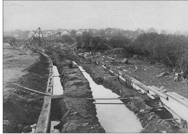
FIGURE 10. Construction of the straightened concrete channel for Alewife Brook in 1911
